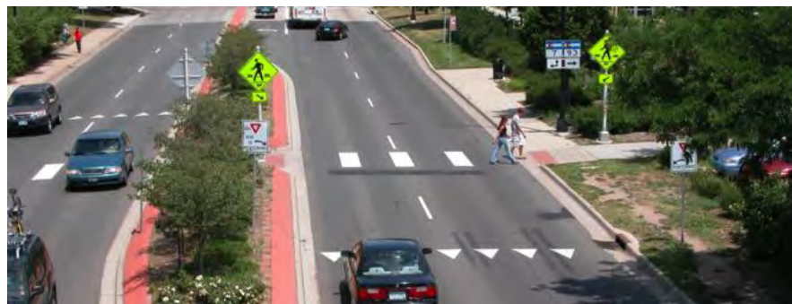
Figure 3 - Rapid Rectangular Flashing Beacon
